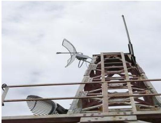
Gambar 3. Transmitter (SBC dan Access Point)
